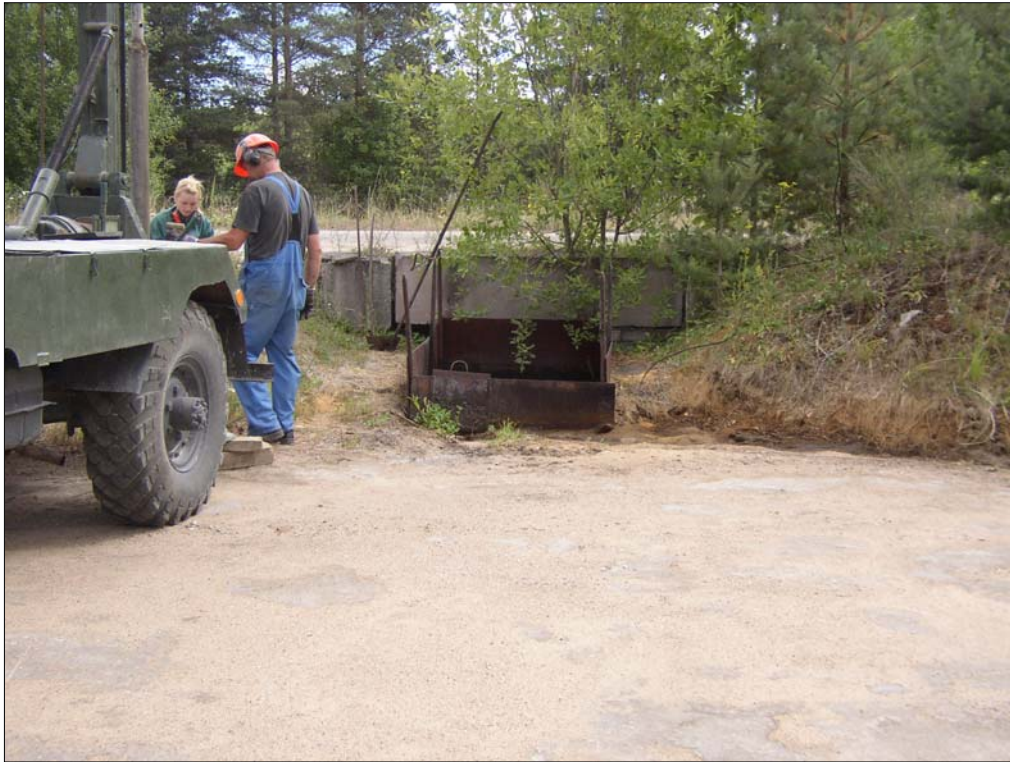
Photo 4008 Location of bore hole 4008, close to oil separator; 21.07.2006
