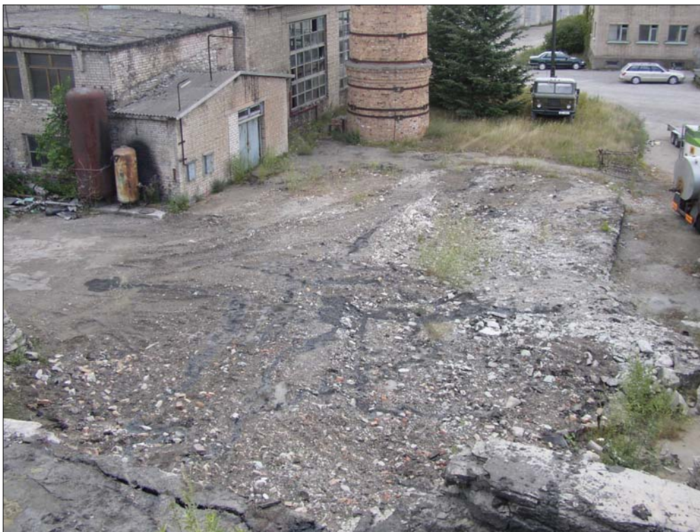
Photo 4000-4. Area of former boilers, covered with naphtha bitumen layer; on the same area is drilled bore hole 4005; 21.07.2006
