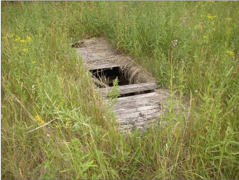
Photo 4000-9. Oil separator close to pond, eastward from ABT; 21.07.2006
