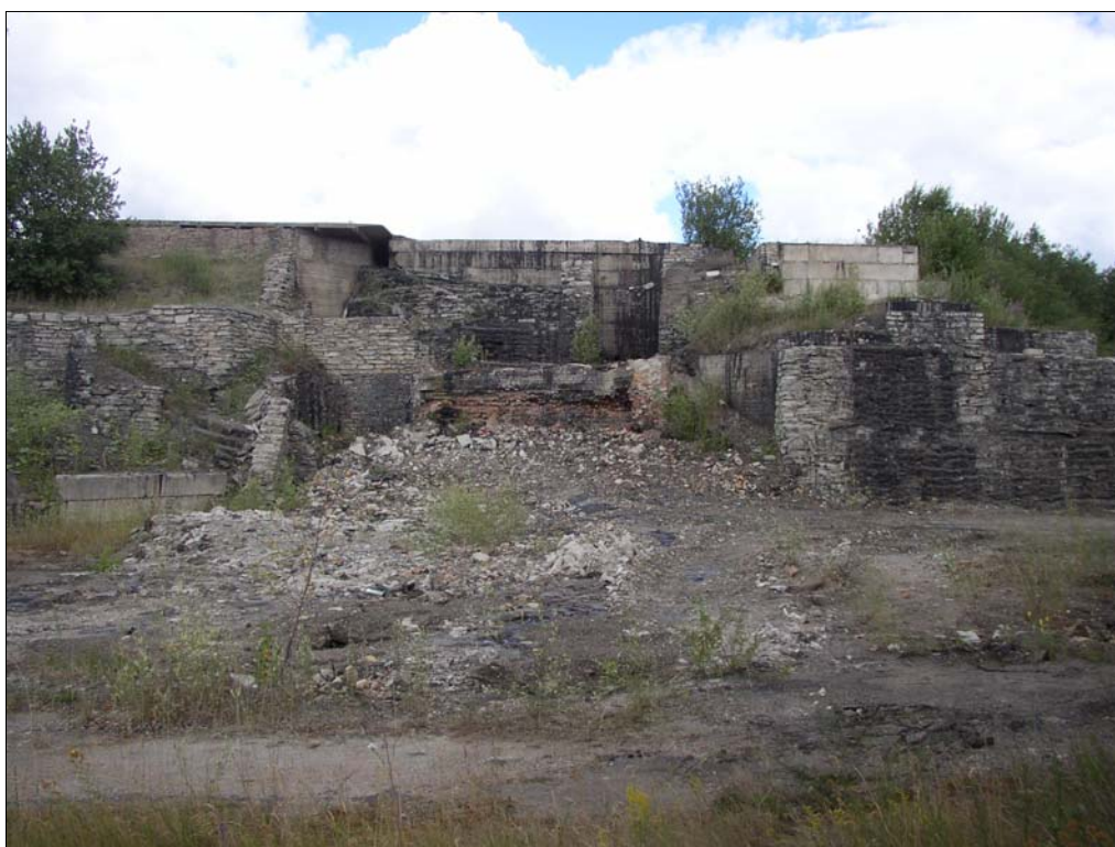
Photo 4000-2. Area of former naphtha bitumen boilers; 21.07.2006
