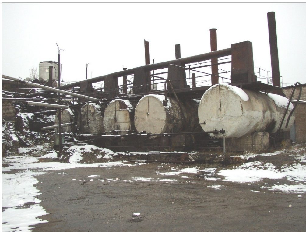
Photo 4000-1. Naphtha bitumen boilers; 15.10.2002
