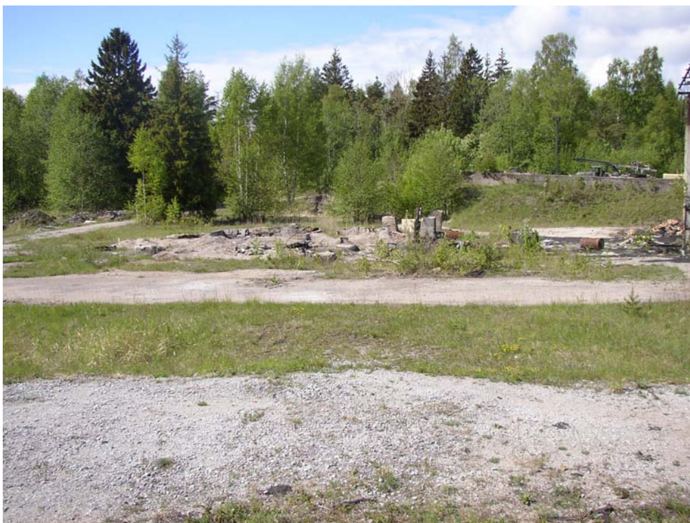
Photo 5701. View to west side of asphalt concrete plant
