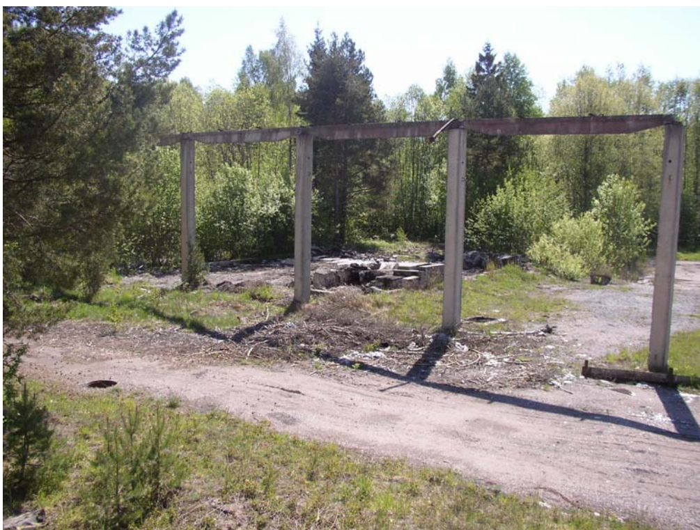
Photo 5702. View to previous fuel storage (close to bore hole 5704 and 5703)
