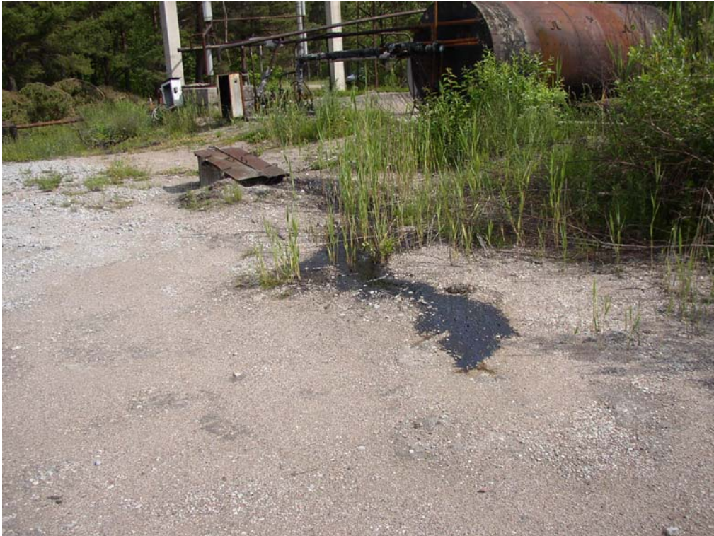
Photo 5707. View to fuel loading system 2003.a (close to bore hole 5703)
