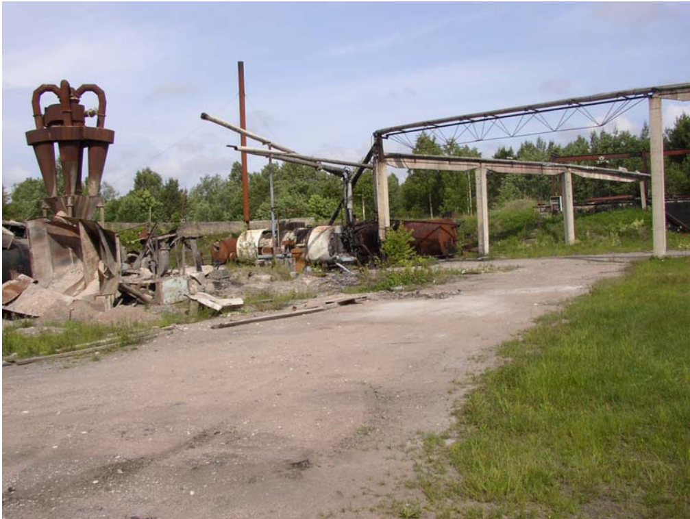
Photo 5705. View from south-west to mixing system 2003.a
