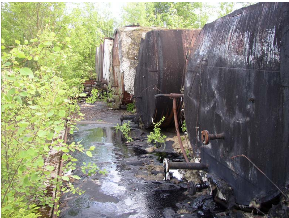
Photo 6600-4. View to open naphtha bitumen tanks and base bath (16.06.2003)
