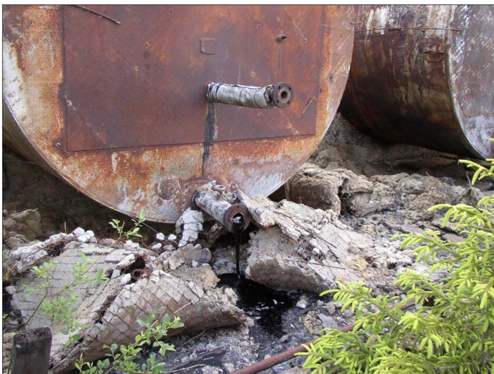
Photo 6600-5 View to spilling naphtha bitumen tanks (16.06.2003)
