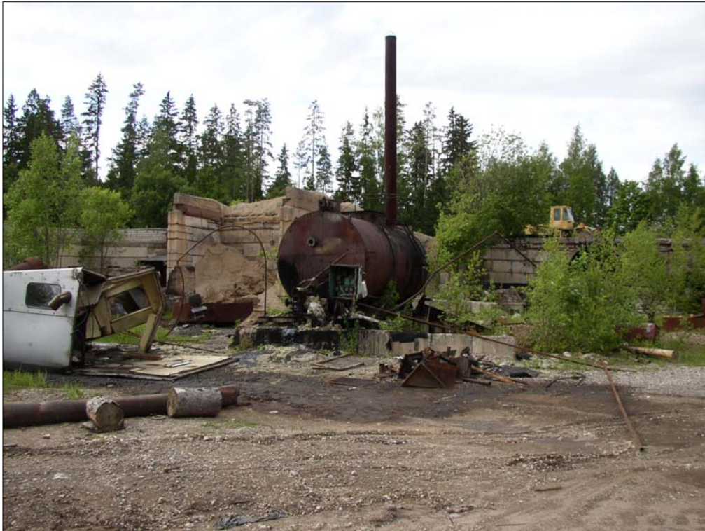
Photo 6600-3. View to bitumen boiler and contaminated ground (16.06.2003)
