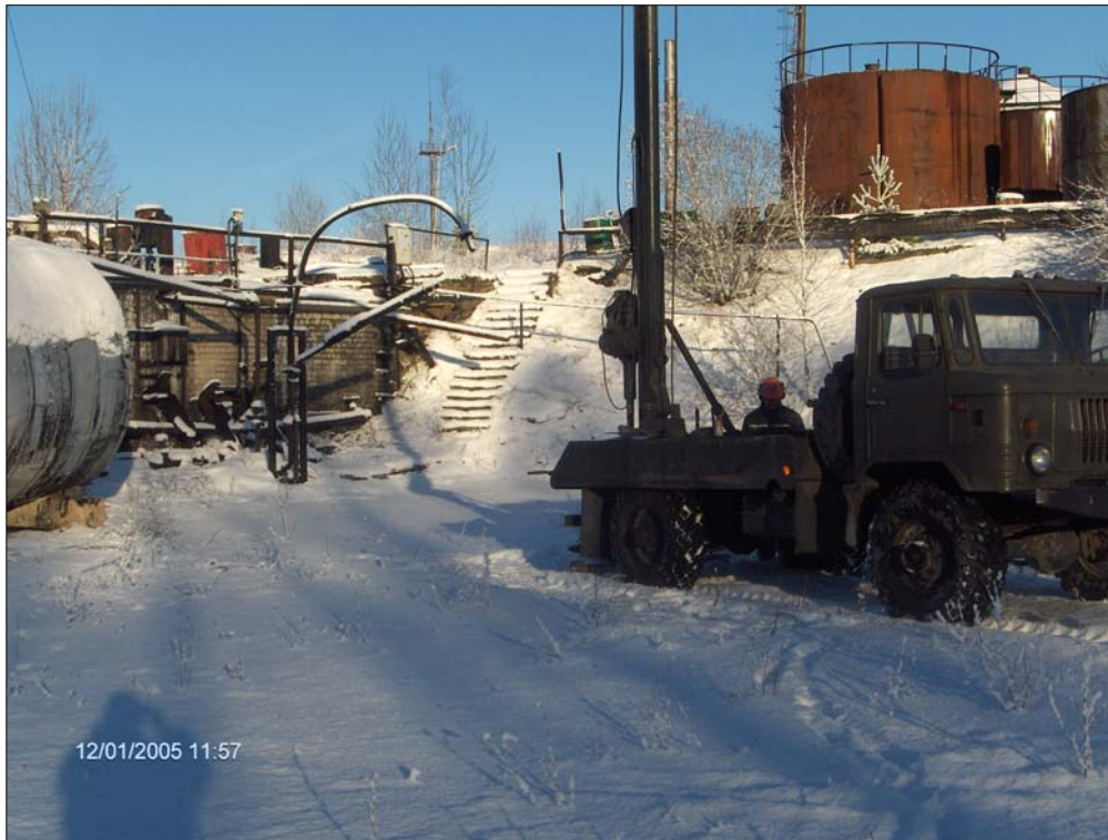
Photo 6520-1. Location of bore hole 6520 – view to north
