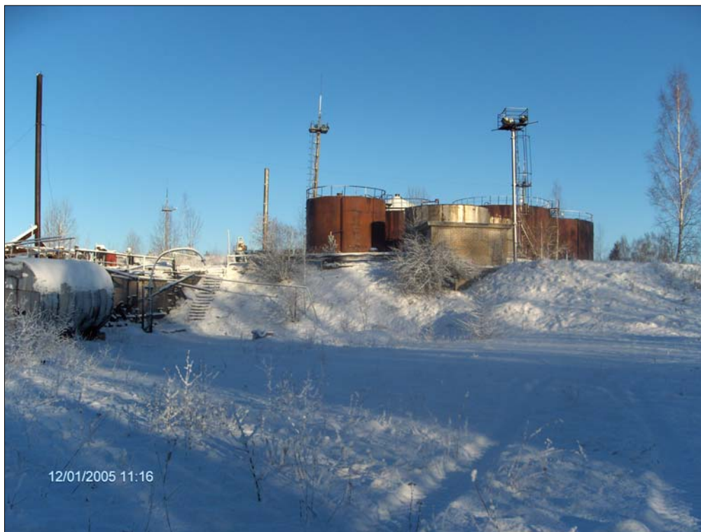
Photo 6500. View to oil shale oil tanks
