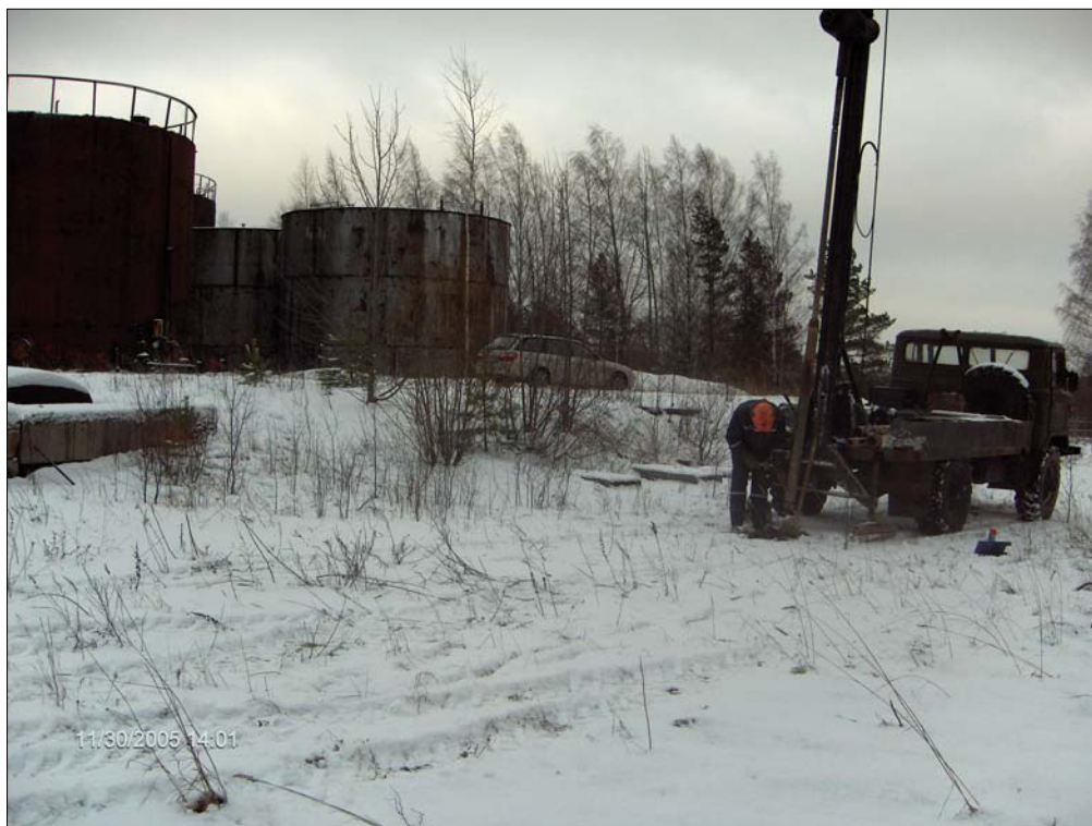
Photo 6512-2. Location of bore hole 6512
