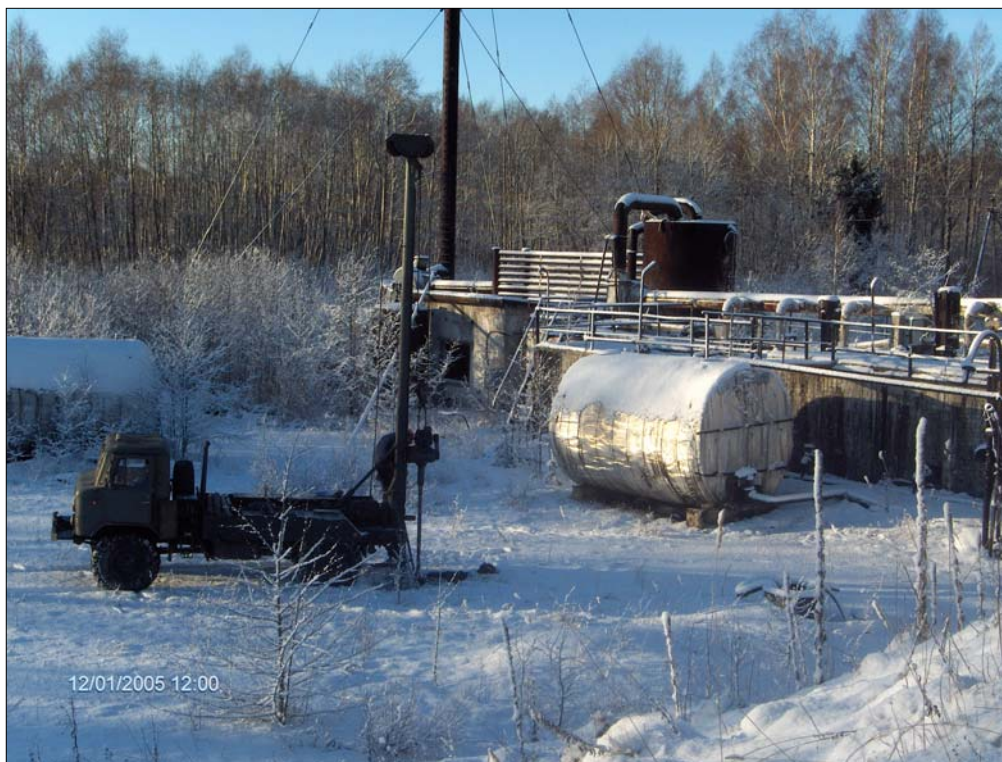
Photo 6520-2. Location of bore hole 6520 – view to north
