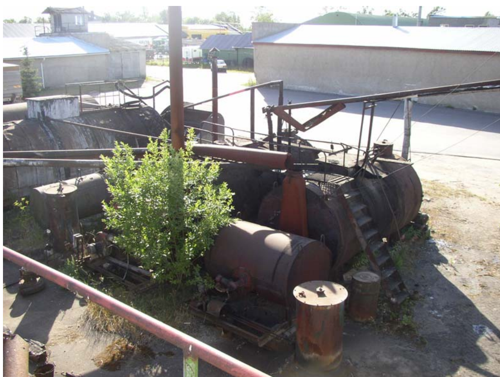
Photo 4700-4. View to the boilers and kettle area; photo 12.07.2006 Surrounding boiler lies bitumen on the ground
