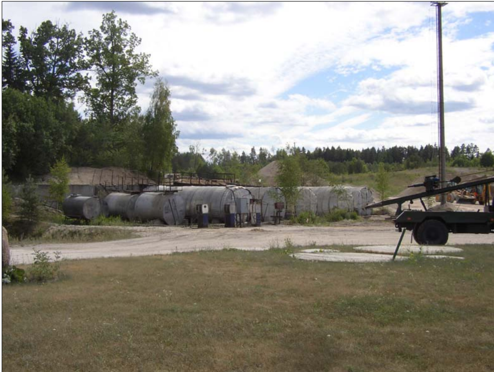
Photo 4500-3. View to the tank area of ABT; photo 17.07.2006
