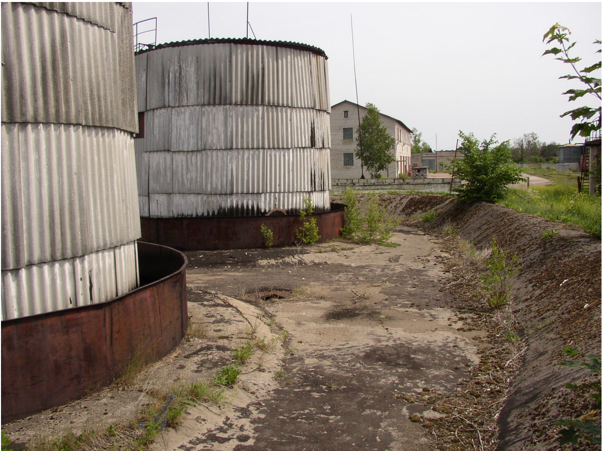
Photo 2 Two a'180 tons tanks
