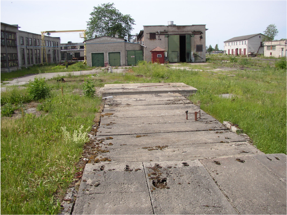
Photo 1 Underground ferroconcrete tank (50 tons) is covered with concrete plates
