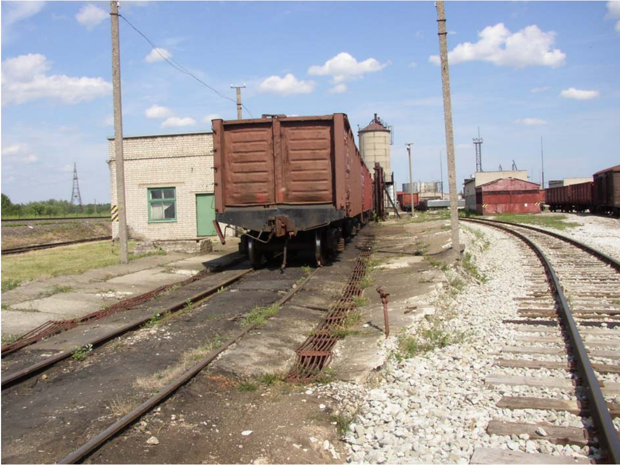
Photo 5 Locomotive wash area and old collecting channels.
