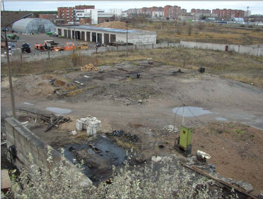
Photo 2900-5 View to the former asphalt mixing unit (oily), farther former boilers area; photo 29.10.2002
