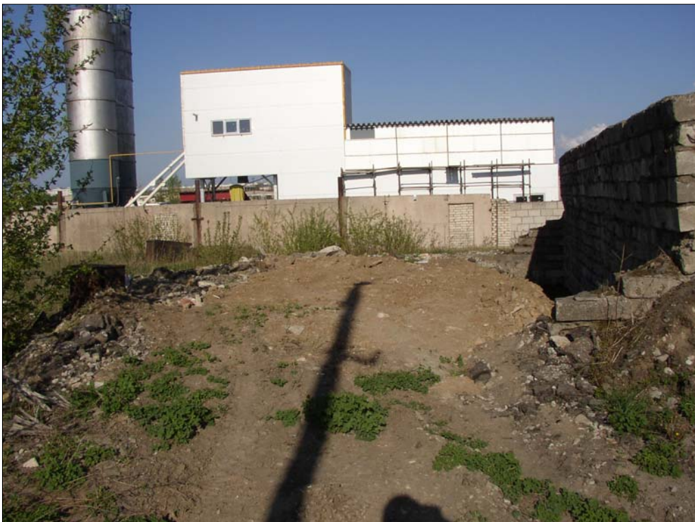
Photo 2900-4. View to the tank area; photo 27.04.2006
