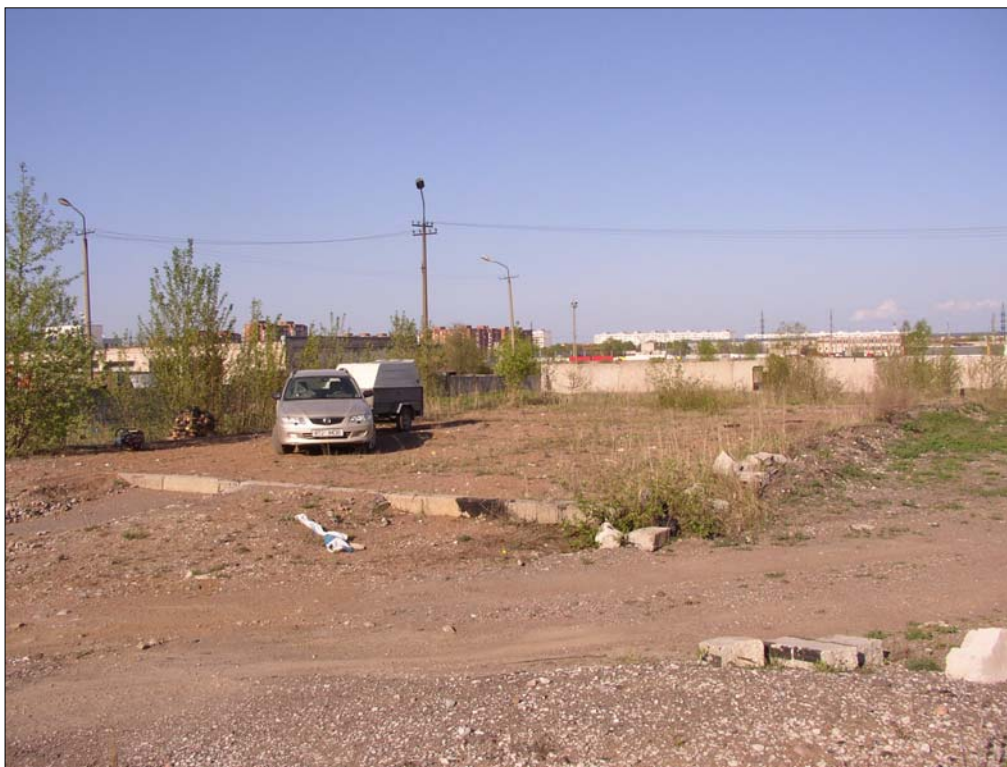
Photo 2900-1. View to the former boilers area; photo 27.04.2006
