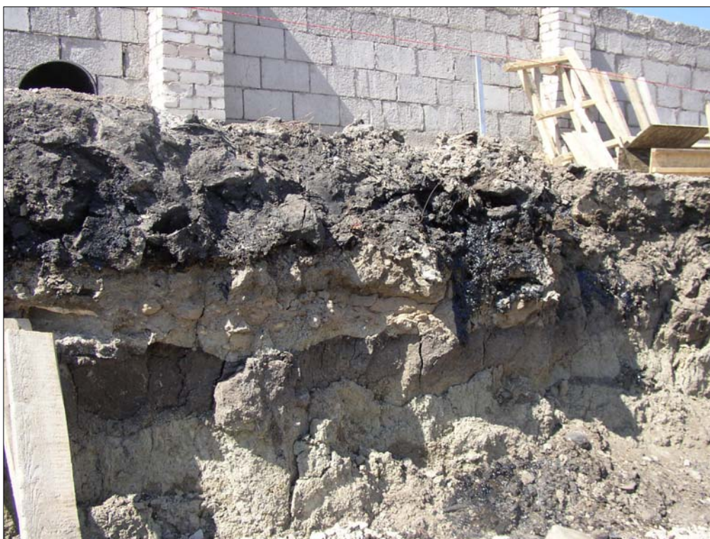
Photo 2900-9. View to hardened bitumen layers of excavated hole on the neighbours territory, located eastwards from ABT; photo 27.04.2006
