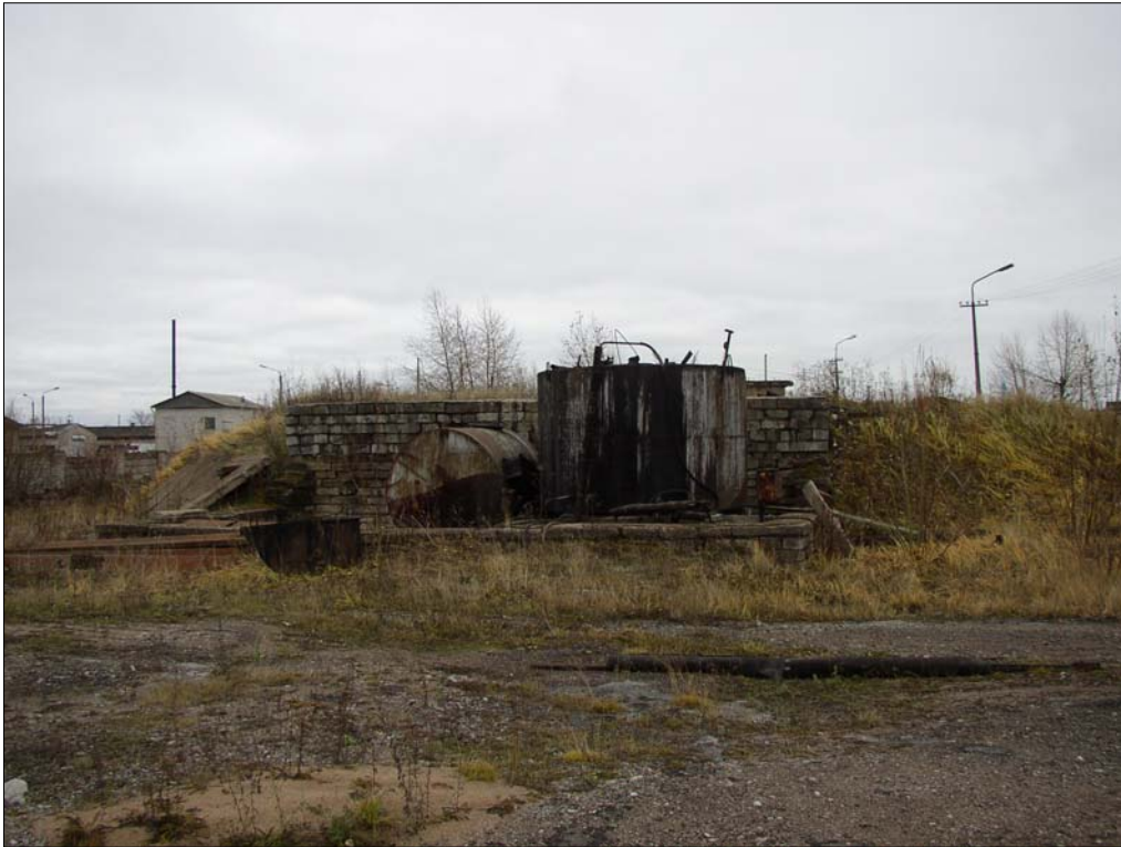
Photo 2900-3. View to the tank area; photo 29.10.2002
