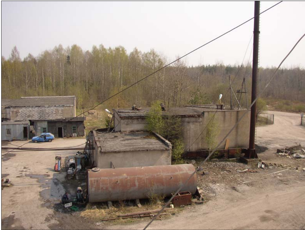
Photo 2500-9. View to boiler house, in front tank for water
