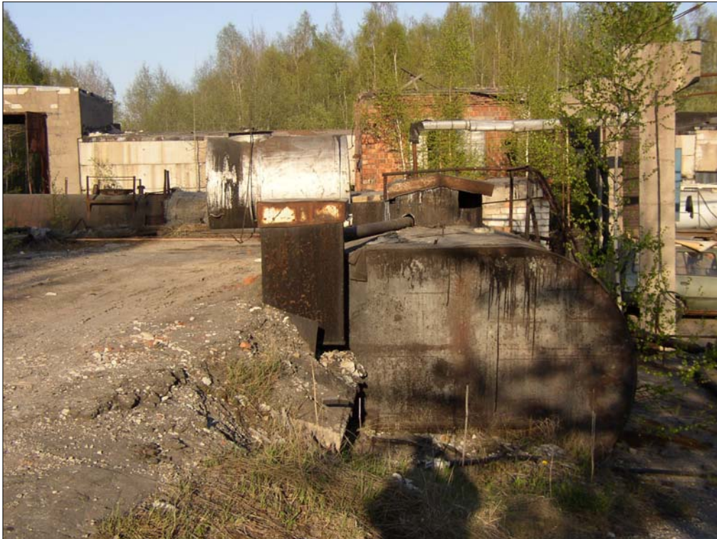
Photo 2500-7. Location of shale oil tank (5) straight on ground
