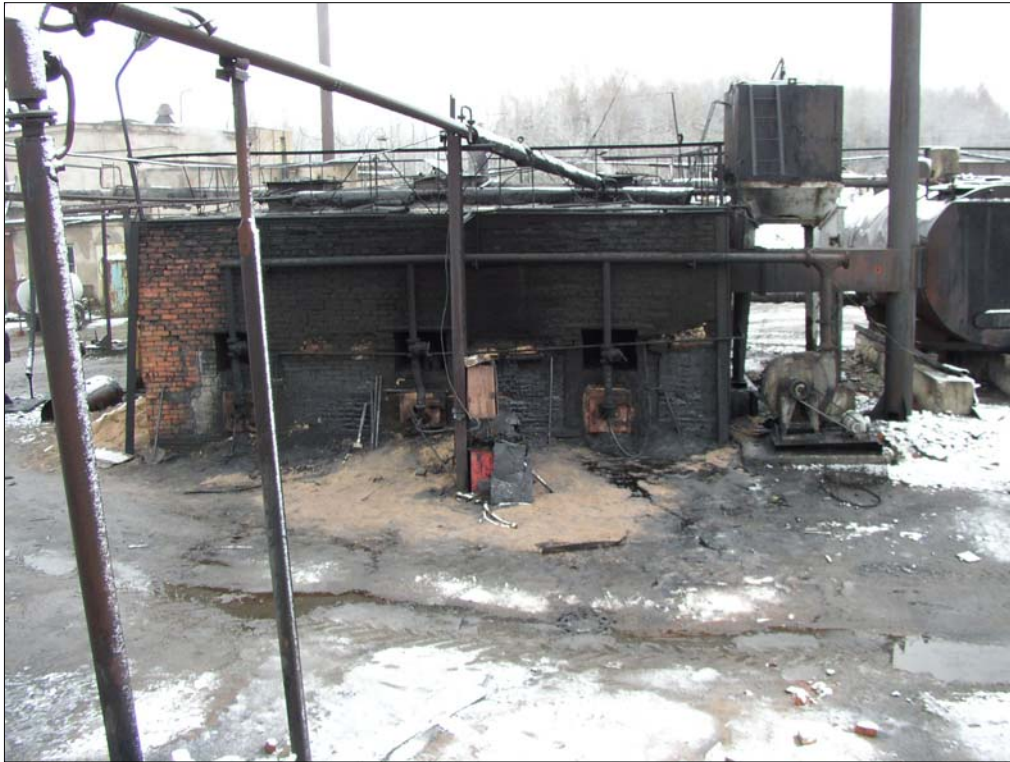
Photo 2500-5 The building with tree old naphtha bitumen boilers (8); photo 30.10.2002
