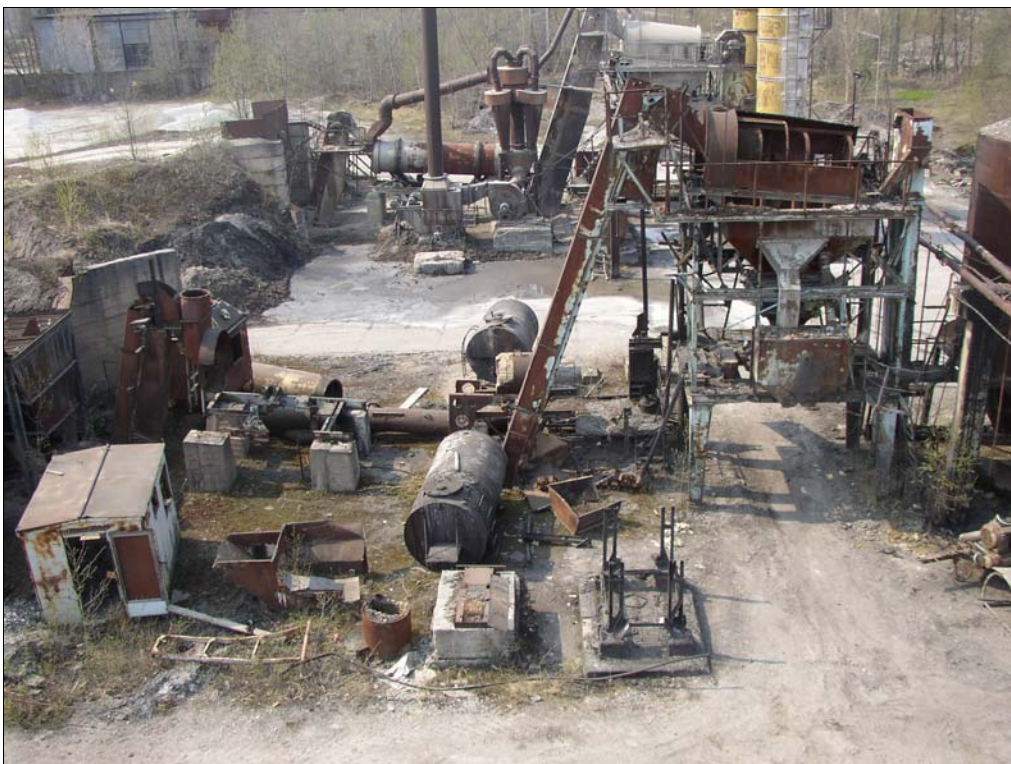
Photo 2500-4. View to the not working part of ABT; the farther unit standing in reserve
