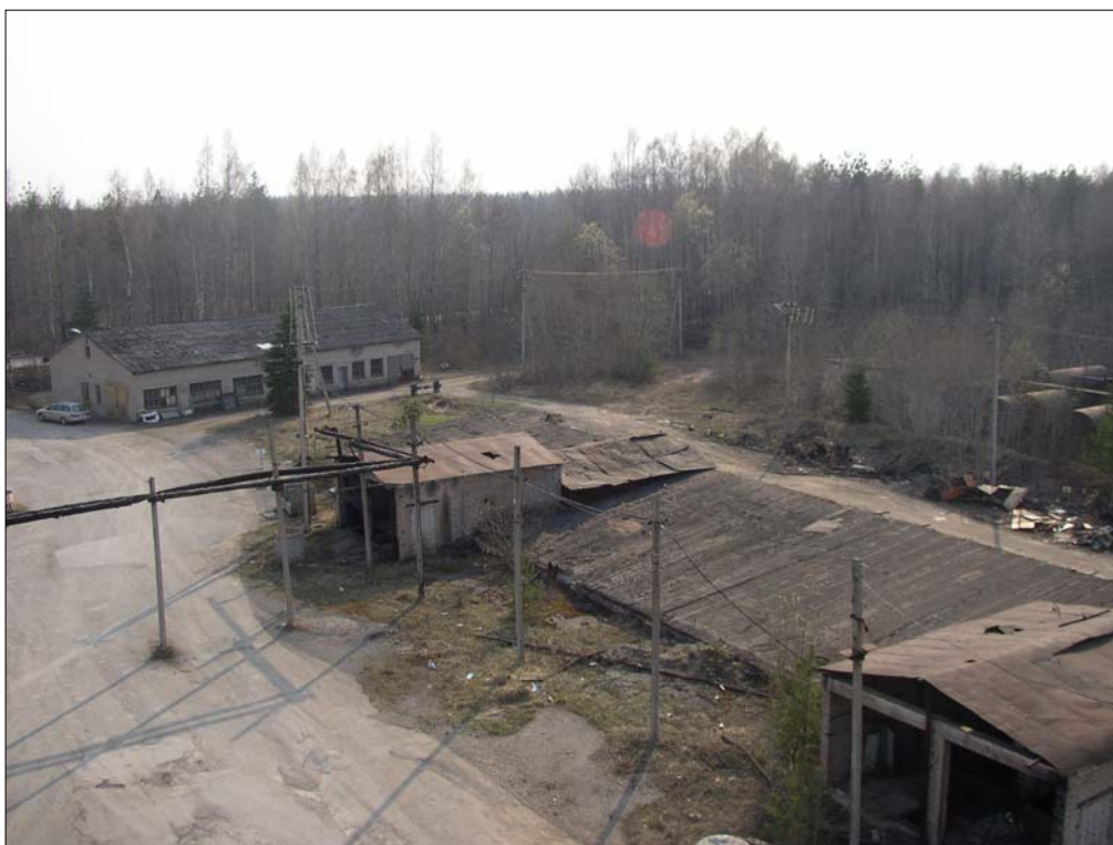
Photo 2400-2. View to naphtha bitumen storage
