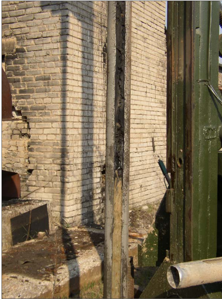
Photo 2423. Contaminated soil in drilling core of bore hole 2423 between 1,1-2,1 m
