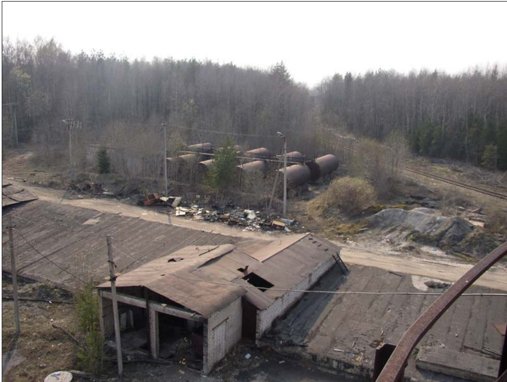
Photo 2400-3. View to naphtha bitumen storage and shale oil tanks
