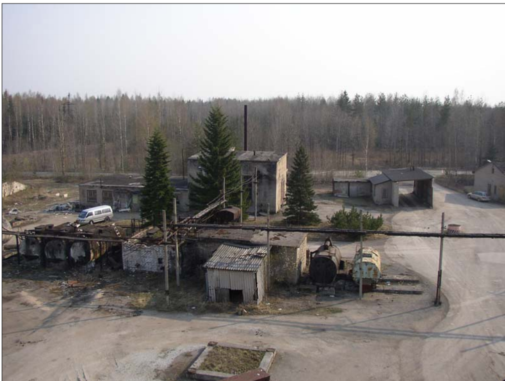
Photo 2400-4. View to old bitumen boilers and boiler house
