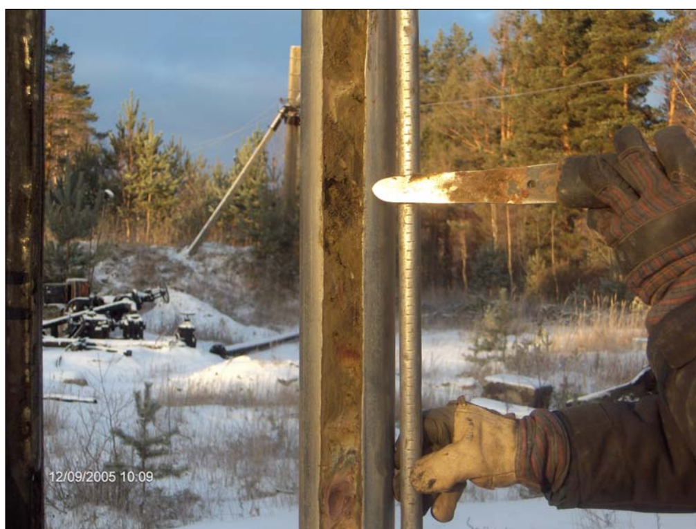
Photo 6912. Oily layer at depth 4,2 m in bore hole 6912
