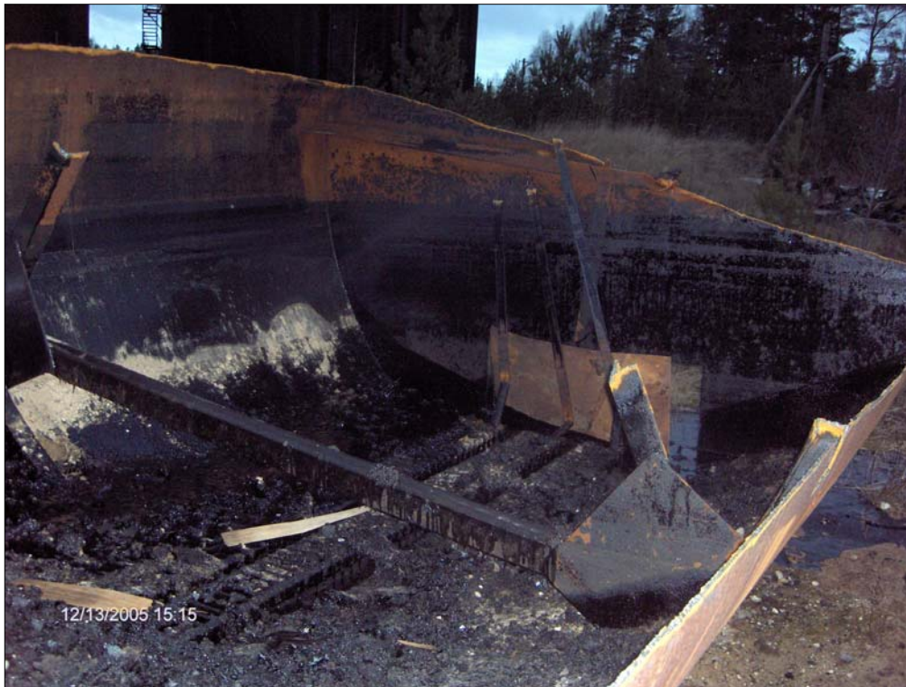
Photo 6900-2. Tank have been cut into pieces close to bore hole 6913
