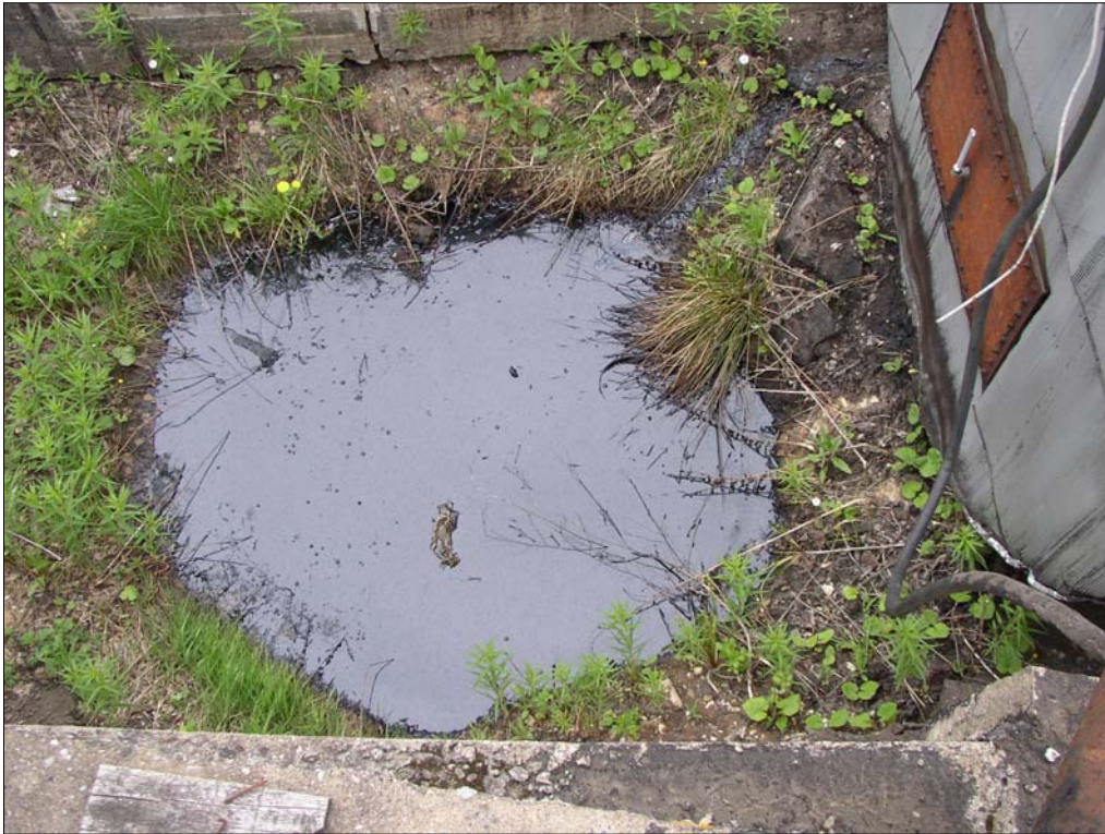
Photo 6900-4. Contamination close to tank 11 (29.05.2003)
