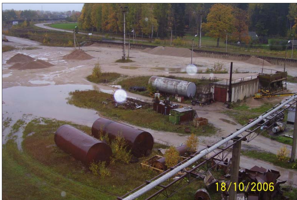
Photo 7300-1. View to ABT territory from tank 1bt north-west
