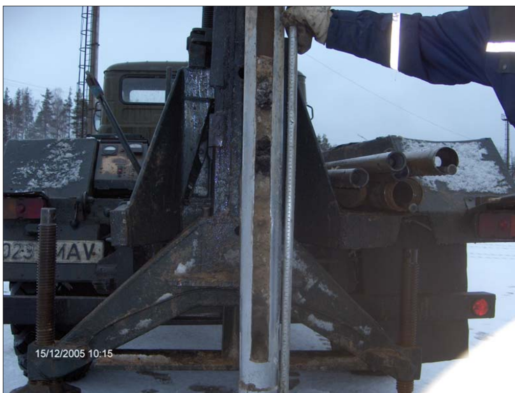
Photo 7304. Drilling core in bore hole 7304 between 0-1,0 m
