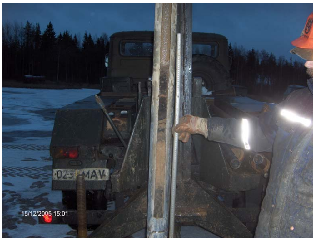
Photo 7312. Drilling core in bore hole 7312 between 2,4-3,3 m
