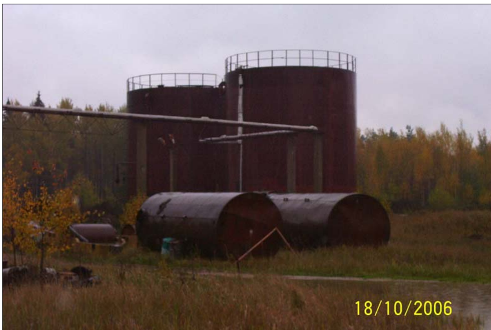
Photo 7300-3. View to tanks 1a and 1b
