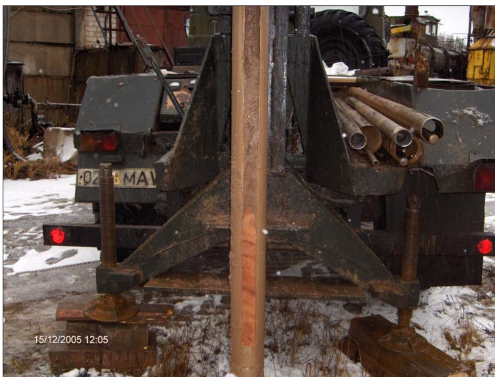
Photo 7306-2. Drilling core in bore hole 7306 between 2,5-4,0 m
