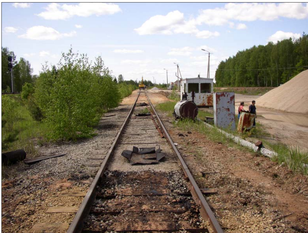
Photo 7300-4. View to railway cisterns loading area (photo 28.05.2003); pollution source 10
