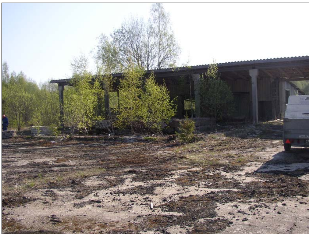
Photo 3401. Building where produced mastic for roofs (close to bore hole 3420)
