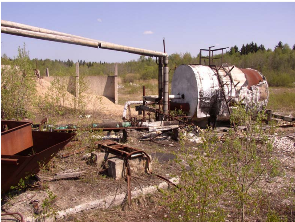
Photo 3404. Boiler close to bore hole 3409
