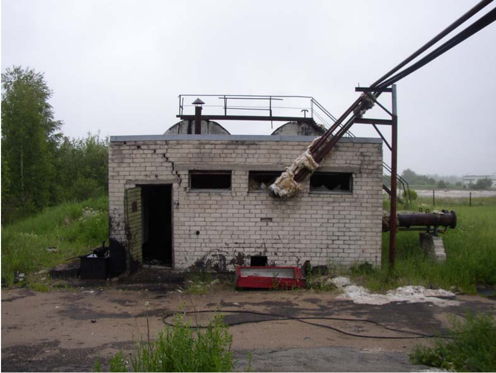
Photo 7003. Boiler house fuel pumping station
