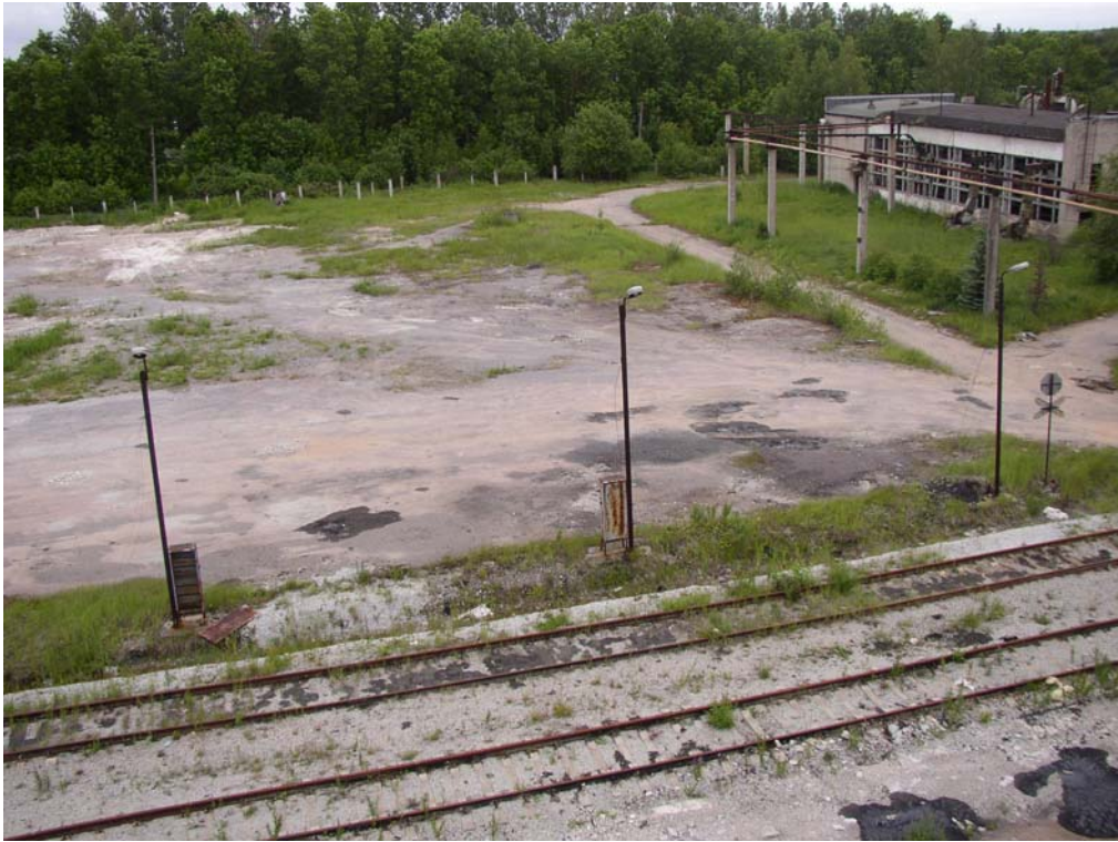
Photo 7001. View to east part of asphalt concrete plant
