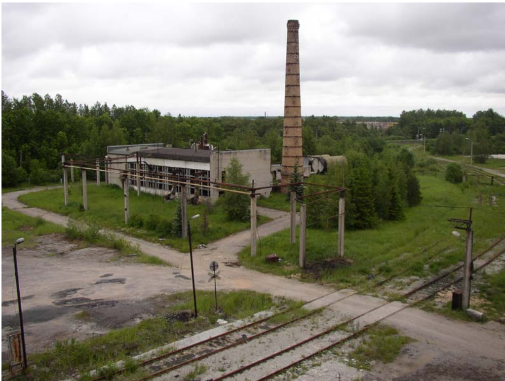
Photo 7002. Boiler house of asphalt concrete plant
