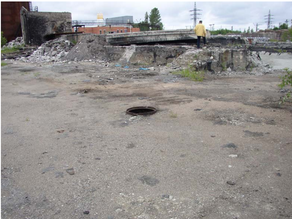
Photo 7006. Underground mazut tank
