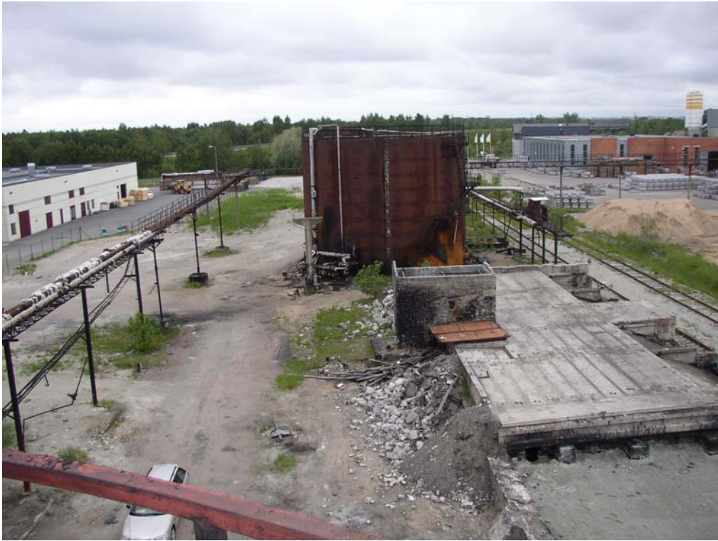
Photo 7005. Fuel tanks and underground mazut tank
