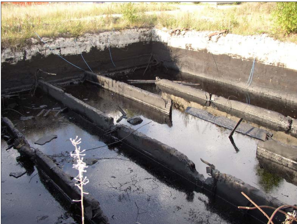
Photo 1500-1. View to the former bilge water separator close to the bore hole 1529; Visible thick layer of oil
