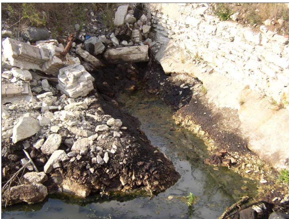
Photo 1500-3. View to the trench for collecting of free phase of oil; on the water is visible thick oil layer and on the slopes of trench is contaminated soil
