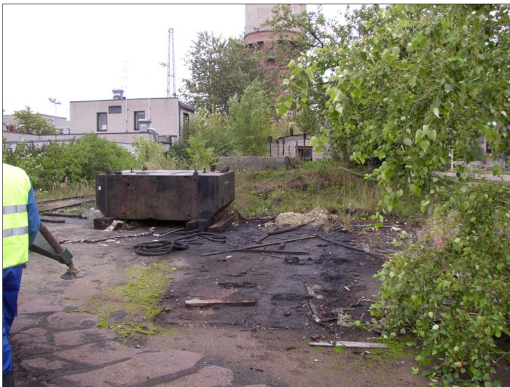
Photo 1201. View to former oil storage from north-west (07.09.2006)
