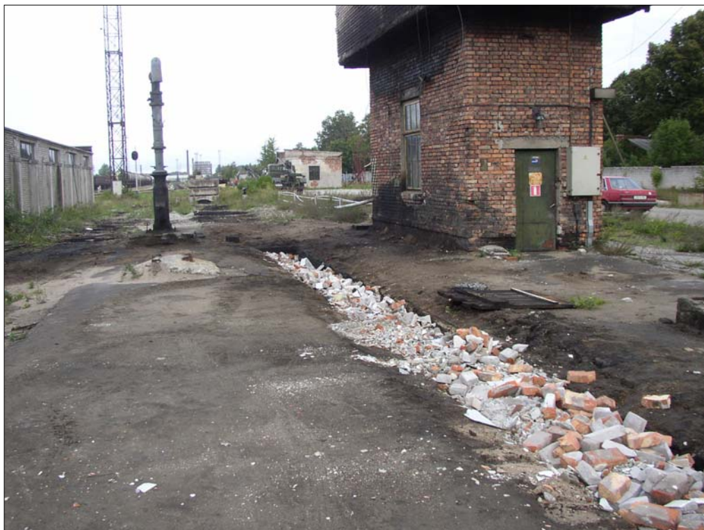
Photo 1206. Probably oily service pits are filled with bricks (07.09.2006)
