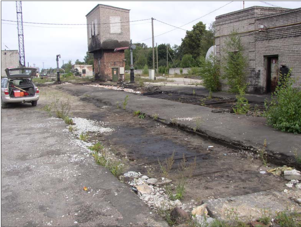
Photo 1205. View to engine service pits; farther is visible building with two fuel tanks inside the 2 nd floor of building; on the walls are visible traces of oil spillages (07.09.2006)
