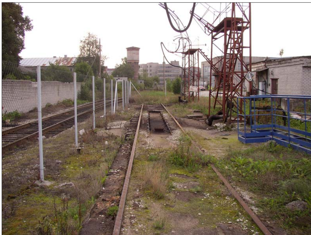
Photo 1204. View to fuel loading area (07.09.2006)
