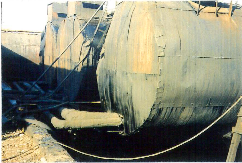
Photo 5. Intermediate Storage Tanks
