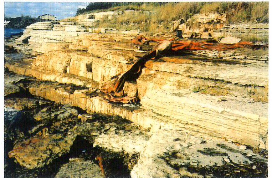
Photo 8. Limestone Embankment, Near Treatment System
