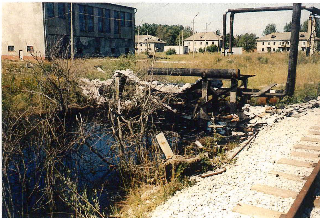
Photo 14. Oil in the drainage ditches on the Western side of the site.
