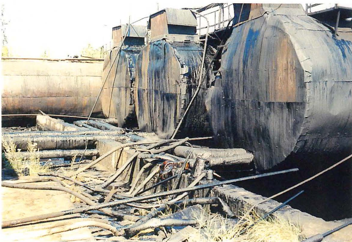
Photo 5. Four 100 m 3 oil tanks in concrete basin (viewed from the south).
