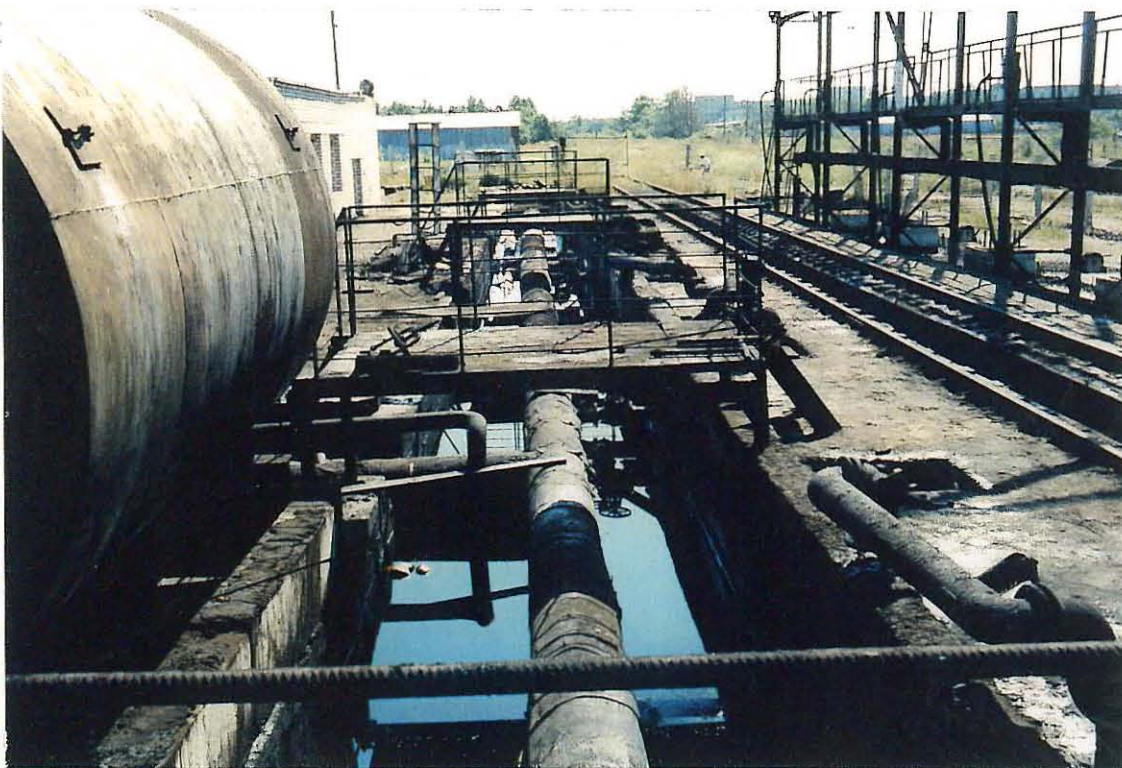
Photo 6. Railway junction for unloading of tank wagons.
