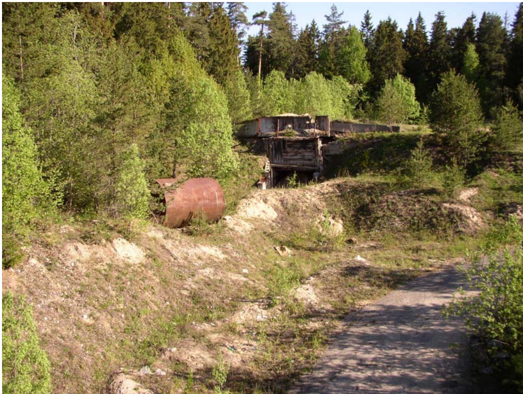
Photo 0201. View from south to asphalt concrete plant (close to bore hole 0201)
